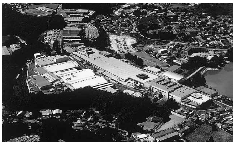
KITZ Nagasaka Plant, Japan
